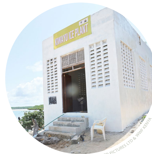
Kiwayu Solar Ice plant
