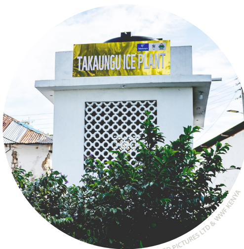
Takaungu Solar Ice plant
